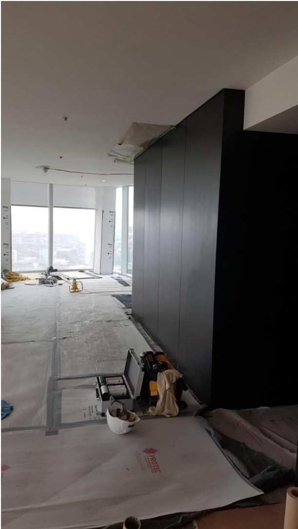
Panelling repaired and recoated
