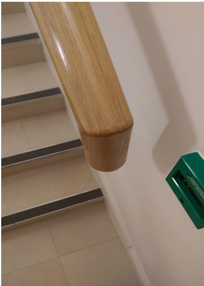
Handrail joint repair rectified
